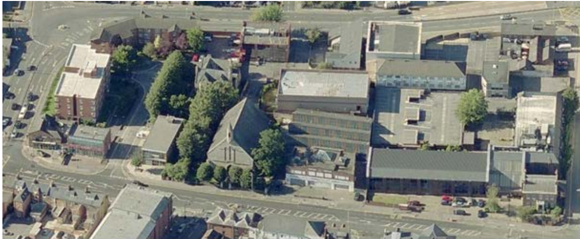
Aerial view looking north.
