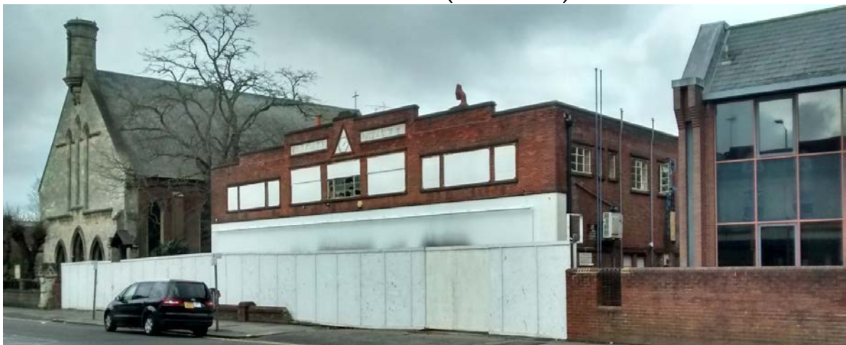
Site photograph dated 05/03/2018.
